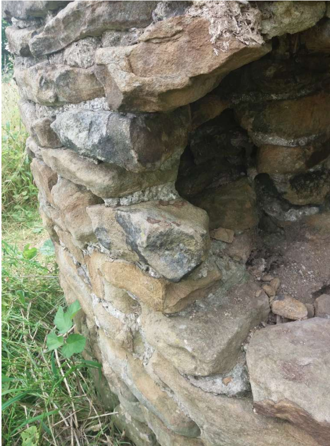
From the north east, showing the wall made of an outer and inner layer of sandstone and rubble fill, with lime mortaring
