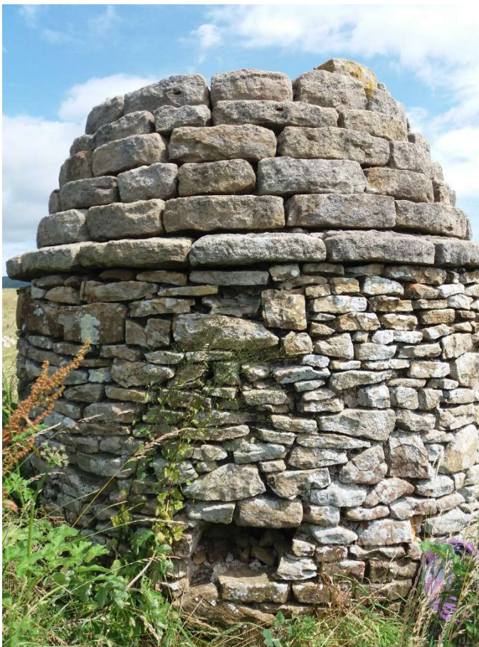
From the south showing wall loss in the outer layer only.
