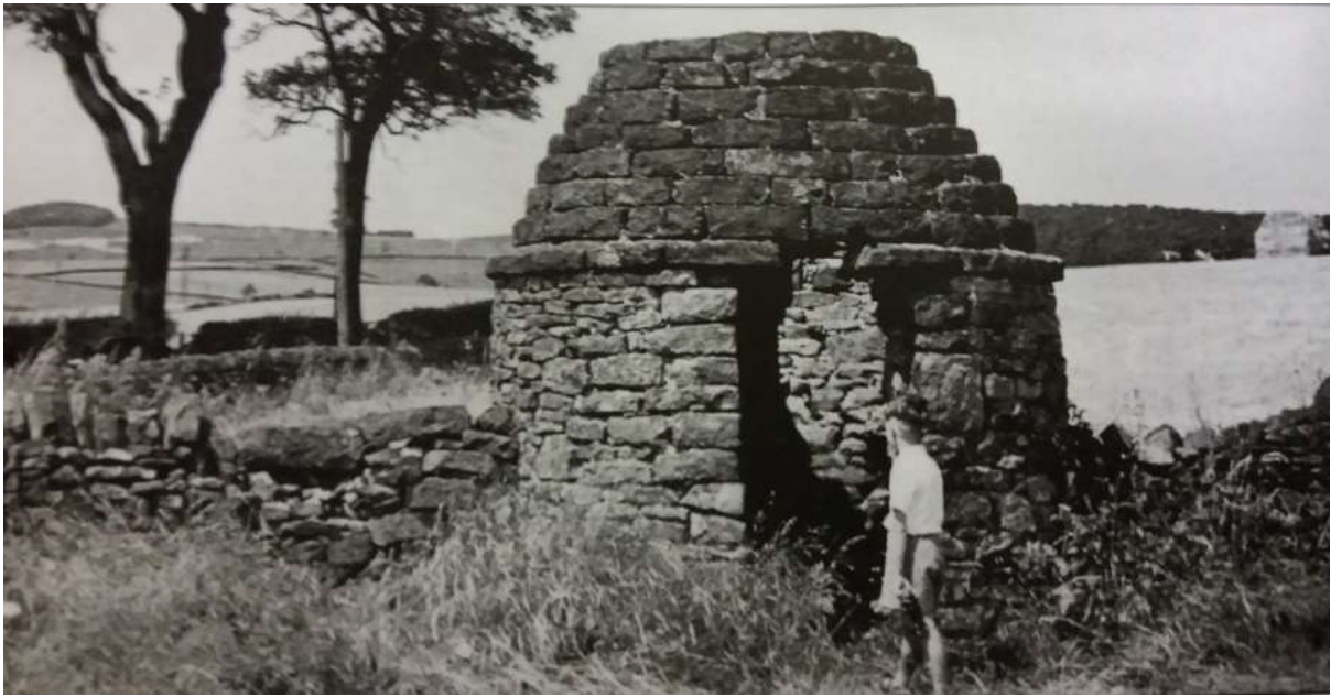
Unknown date (first part of 1900s?) showing the roof with seven courses of stone and with keystone absent and showing field walls on either side. Frank Rodgers. (N.B. I have been unable to contact the photographer to ask for permission to use this photograph or to establish a more definite date.)
