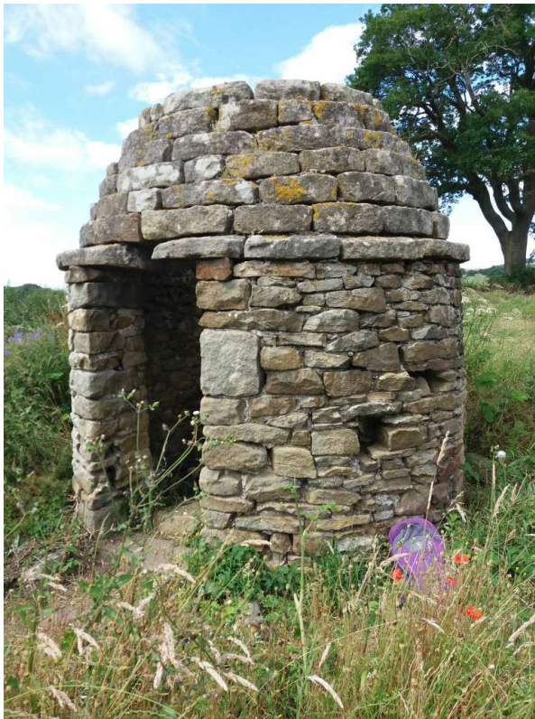
From the north east showing two areas of wall loss and the stone sill of the doorway.
